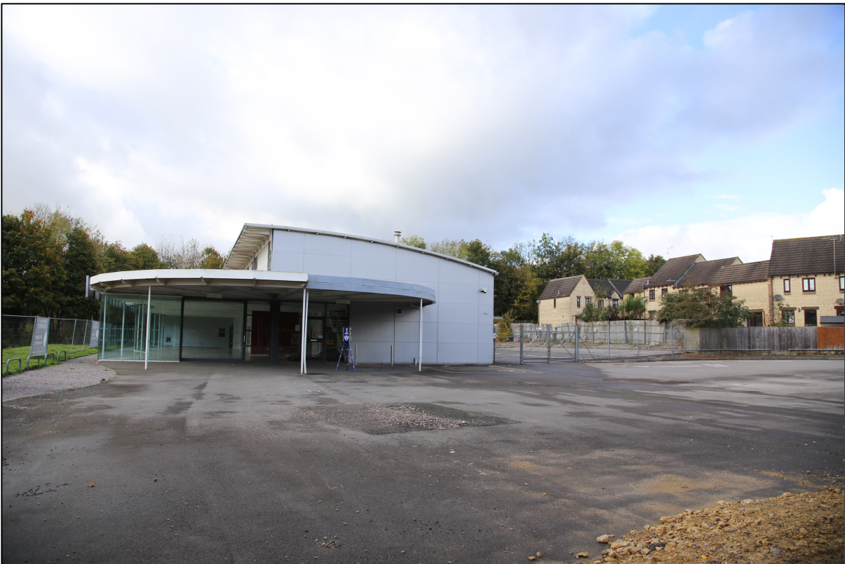
View of existing building and car parking
