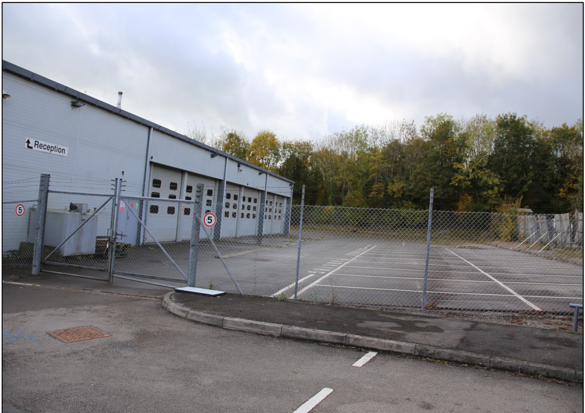
View of existing yard
