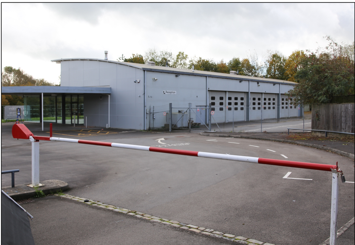
View of existing access with barrier
